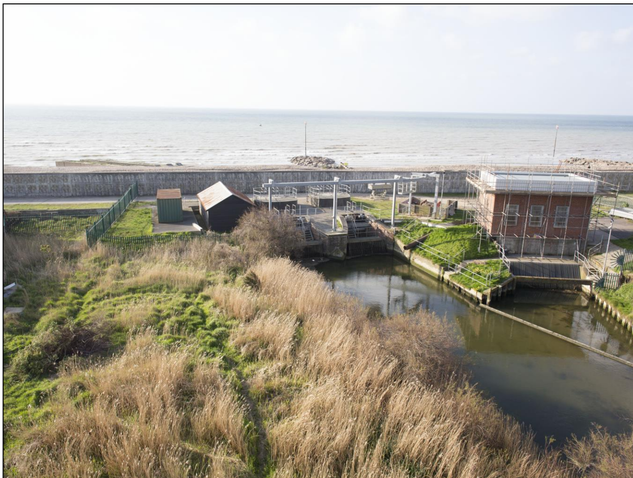
Tidal sluice and pumping station on the Aldingbourne Rife at Felpham
